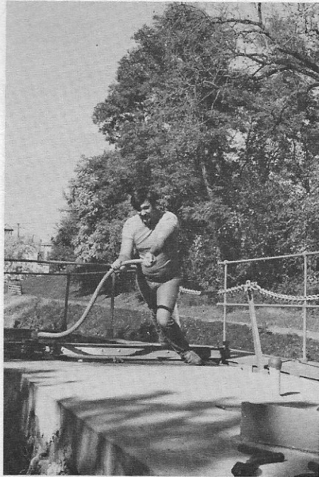
Only muscle power is used in the operation of Muskingum River locks.
