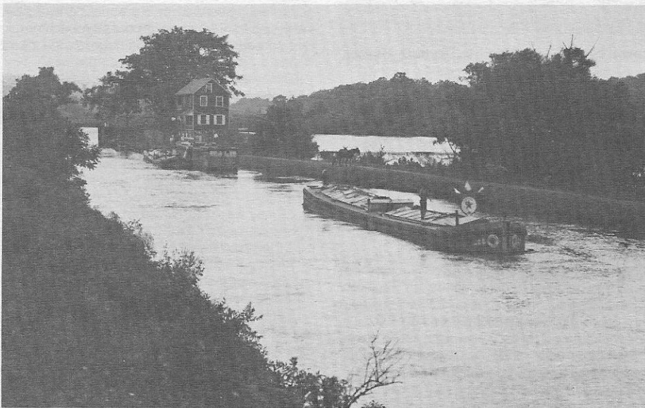
This old photo, which was found in the files of Alvin F. Harlow, shows the section of the Lehigh Canal on which we made our boat trip during the PCS Tour, the way it looked about 1920. The old dam, which fed water into the three-mile section of the Lehigh from this point down to Easton, may be seen at the upper center. (Courtesy of Walter Meseck.)
