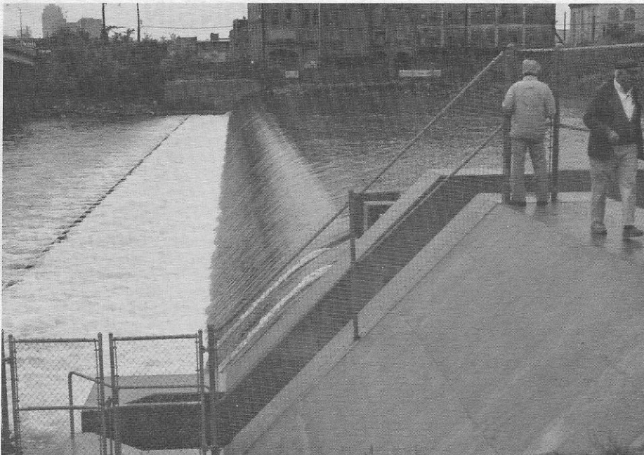
The recently rebuilt Lehigh River Dam at Allentown, which feeds water into the Lehigh Canal at this point. Some of the PCS members are shown standing on the downstream end of the Fish-Ladder.
