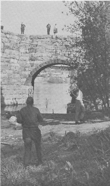
View through the archway on the Delaware River at Phillipsburg, New Jersey where the westernmost Plane on the Morris Canal picked up Lehigh Canal Boats from Easton, Pa. across the river. The City of Easton can be seen through the arch. (Photo by Bill Shank.)
