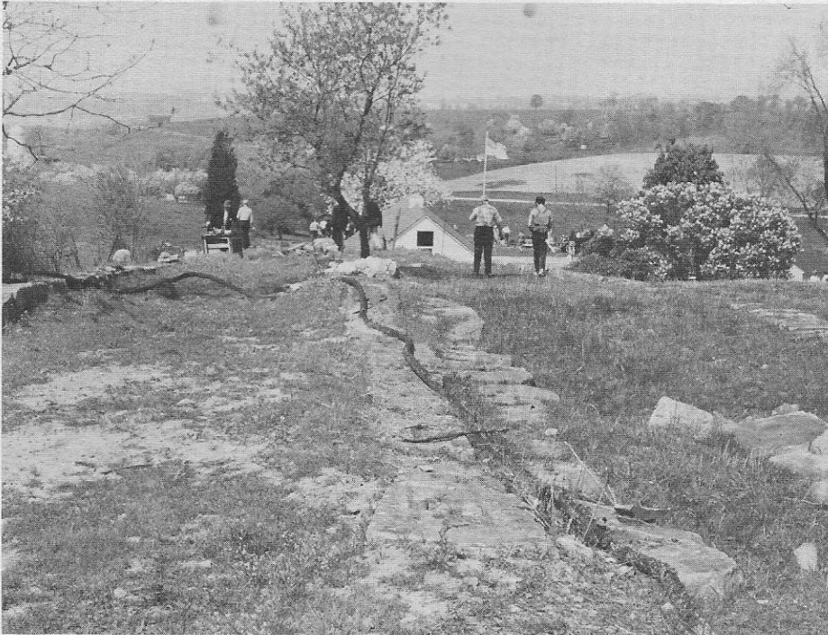
A view made over "the hump" of Inclined Plane Nine West. Note the old twisted wire cable from the plane in the foreground. Jim Lee's home (a former lock-keepers house) can be seen, downhill, at the center of the picture. (Photo by Bill Shank.)
