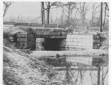
Remains of Blackstone Canal Lock at Church Street, Northboro, Massachusetts. Lower gate recesses are under the bridge. (Photo by Dave Barber. 3/12/88.)
