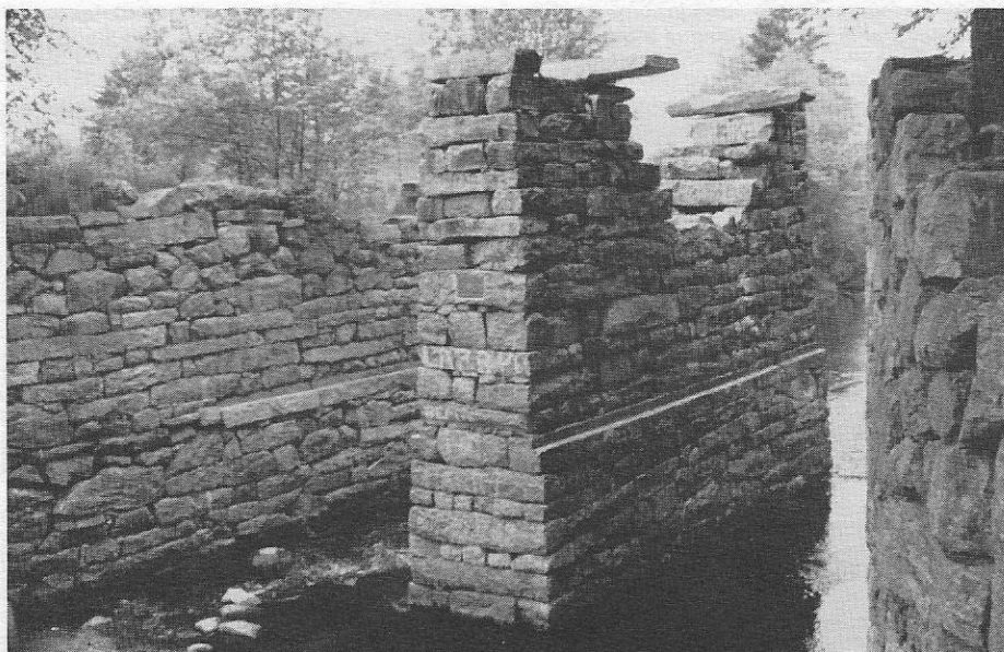
Shawsheen Aqueduct/abutments and center pier on the Middlesex Canal (Photo by E.S. Andersen.)
