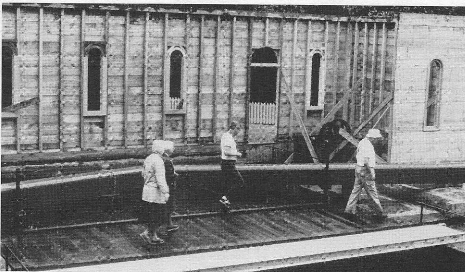
Pawtucket Canal toll building reconstruction, by upper Guard Lock.
