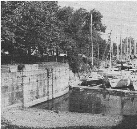
Entrance Lock to the Second Welland Canal at Port Dalhousie. Built in 1841, it was extra large to allow larger vessels to reach St. Catharines from Lake Ontario. Balance of the Second Canal locks were smaller. (Russell photo.)
