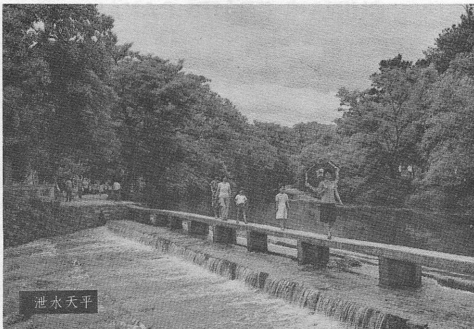
A water-level control dam discharging surplus water from the Lingqu Canal. A pedestrian walkwalk makes the connection between two sections of the old towpath.
