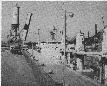
An ocean-going vessel in Lock Number Four near St. Catharines. Note the tall "surge tower" on the left, which provides water for power generation on this section of the Welland Canal. (Russell photo.)
