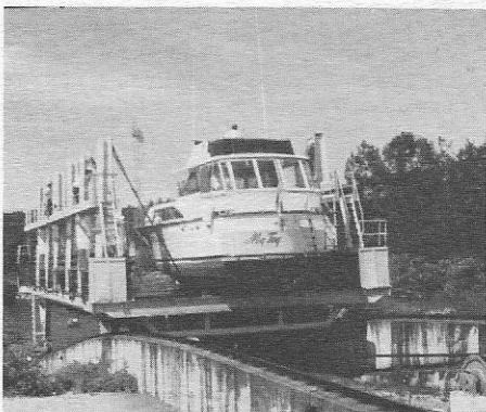
"Big Chute", with a boat in the cradle going "over the hump" on the way down to the lower level.
