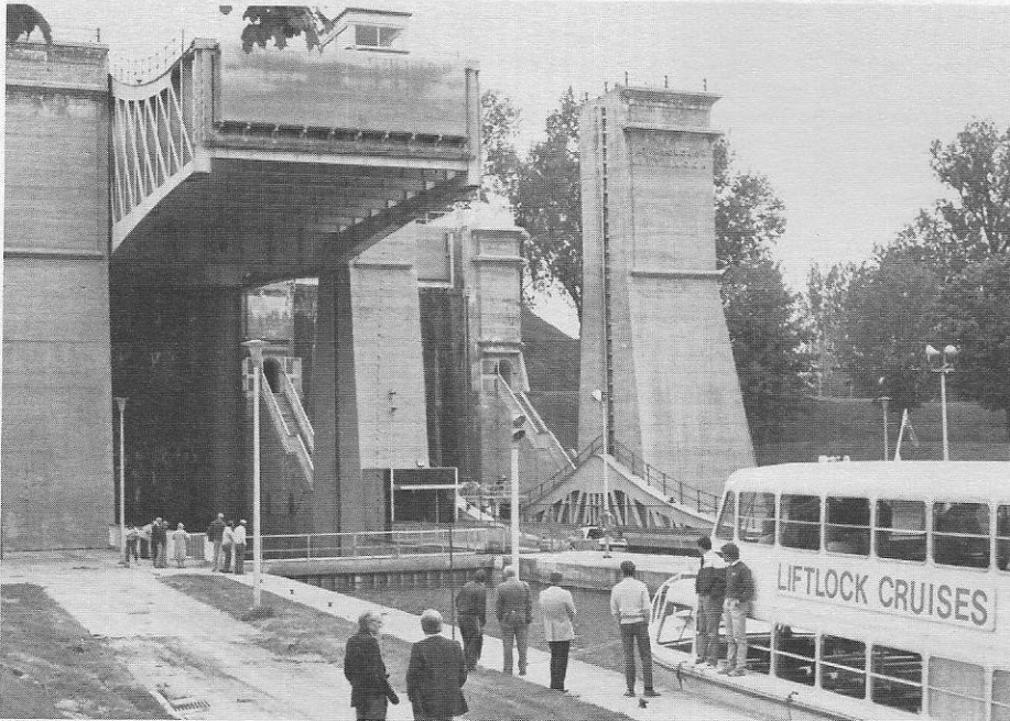
The world's highest hydraulic lift locks at Peterborough.
