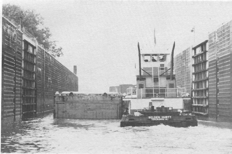
A tow leaving Oliver Lock at Tuscaloosa, mile 338.1.
