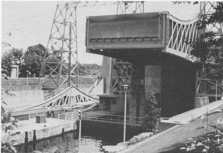
The hydraulic lift locks at Kirkfield.
