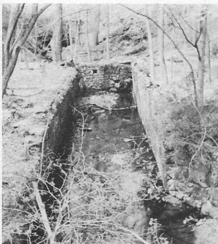
At Rosendale this "Canal siding" ran off the main channel directly into the Snyder cement works to allow canal boats to unload coal for the kilns and pick up bags of newly-made cement. (Russell photo)
