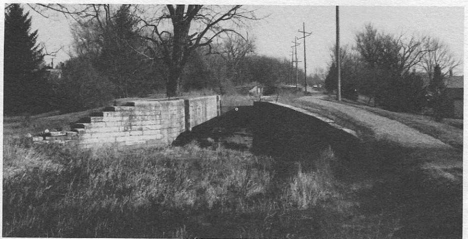
Photo sent us by Gerald Hulslander of Marseilles, Illinois showing the two lock ruins of the old Illinois and Michigan Canal in that city. Gerald reports that the area has been kept tidy by the local citizenry, and the old towpath is maintained in good condition for hiking and biking.
