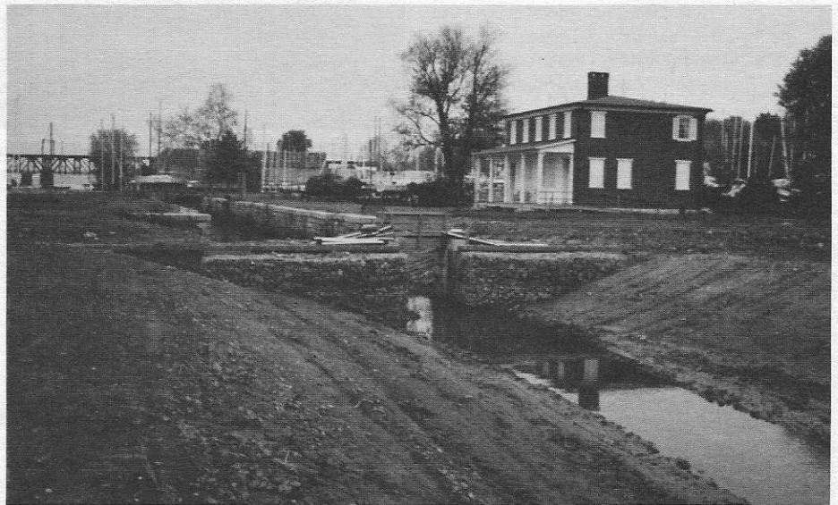
General view of the south end of the shad-holding pond (foreground) the pond-level control weir (center) and the restored tidewater lock and Museum in the background.
