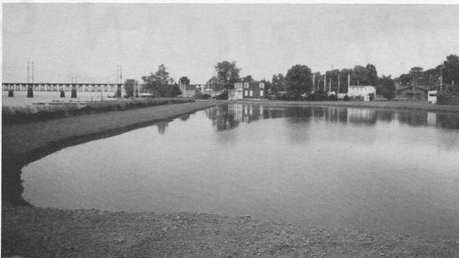
Shad-holding canal basin at Havre de Grace, Maryland filled with water. (See Issue Number 73 of American Canals.) Old towpath on the left; Lock-keepers House (now a Museum) in the center background, adjacent to the outlet lock from the basin.
