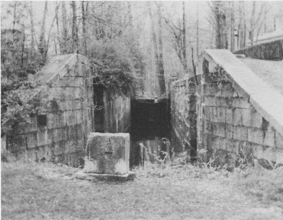
Lock Number 16 on the D. & H. Canal at High Falls, New York. This was one of a series of five locks (Numbers 16-20) that took the canal over a hill. They are part of a re-building of the canal which occurred in 1848-50, by-passing the original right-of-way. (Russell photo.)
