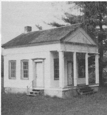
One of two surviving toll houses on the D. & H. Canal. This 150-year old building is located at Ellenville, New York, but has been moved from its original location when the canal bed was filled in for a local street in the 1920's. (Russell photo.)
