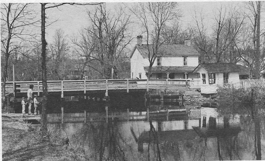
Delaware and Raritan Canal State Park: Blackwell's Mills Bridgetender's House and Station. Photo by J. Amon, 1989.
