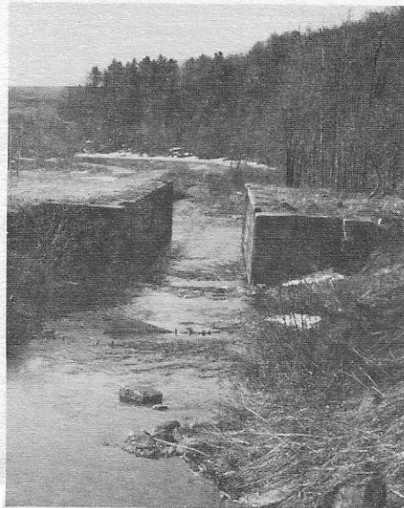
Black River Canal, Lock 64—top of the Boonville Gorge looking south. The canal here began a steep descent from the summit level down to the Mohawk River valley carrying water tapped from the Adirondack foothills ultimately to the Erie Canal at Rome.
