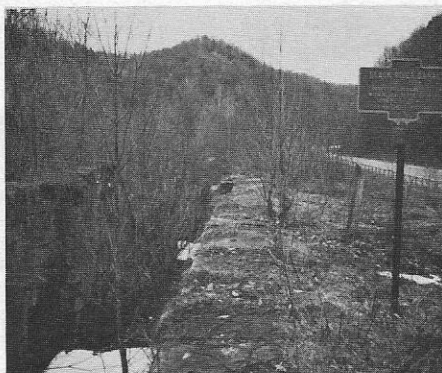
Black River Canal Combine Lock—one of several sets of combines on this "mountain goat" canal which had 108 locks compressed into a mere 35 miles as it surmounted the divide between the Mohawk and Black River valleys. The sign reads, "Black River Canal—1837-1922—Connected Mohawk Valley with Black River country opening up 90 miles of navigable waterway."
