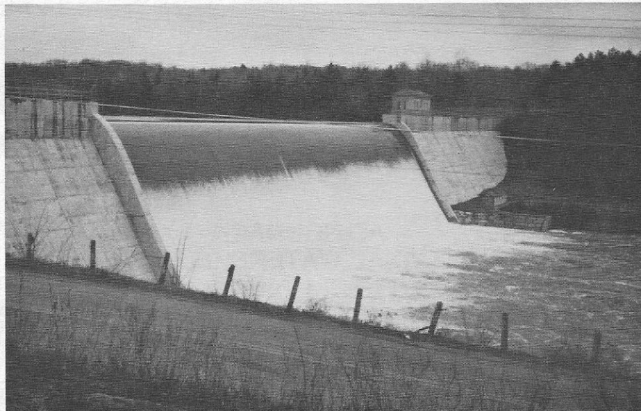
Delta Dam on the Mohawk River—a few miles north of Rome, this dam impounds the drainage from the western Adirondack foothills for today's Barge Canal. It replaced the old water delivery system by way of the now-abandoned Black River Canal.
