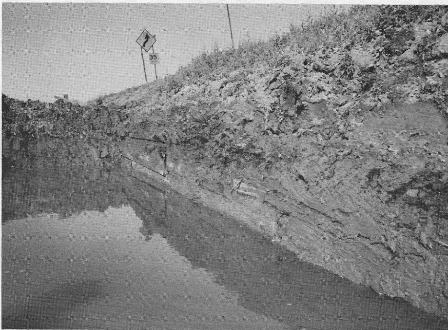
Two views of Gronauer Lock #2, unearthed recently by a highway construction crew working on an interchange east of Fort Wayne, Indiana. Some of the old wood timbers are visible in these views.
