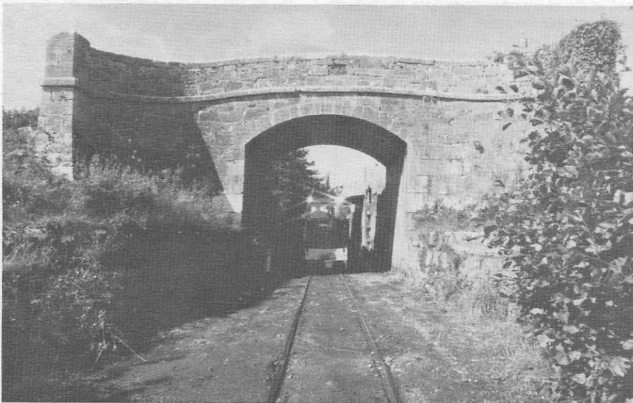
Here the rail line passes through the arch of an old canal bridge. The Irish Peat Board operates 800 miles of such railway to transport the fuel to power plants. Similar lines cross over the Grand Canal main route at several points on moveable bridges.
