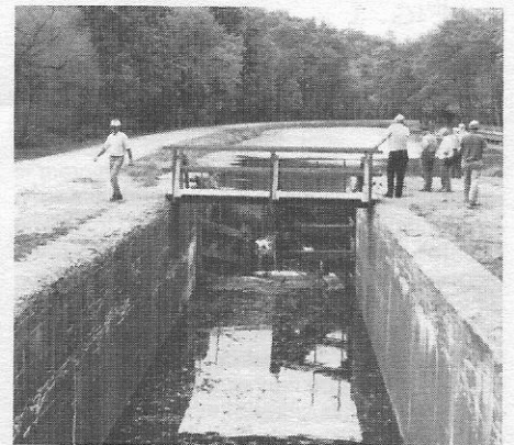
A watered section of the canal near Town Creek Aqueduct. The decrepit lock gates have been supplemented by a weir to hold back the water above the lock.
