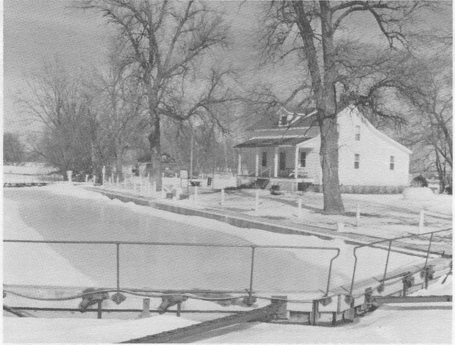
The Eureka Lock and locktender's house near Oshkosh are the only lock facilities still in use on the Upper Fox River. The lock here was closed in 1951 but reopened in 1958, and is operated seasonally by the Berlin Boat Club. The lock and house are listed in the National Register of Historic Places.
