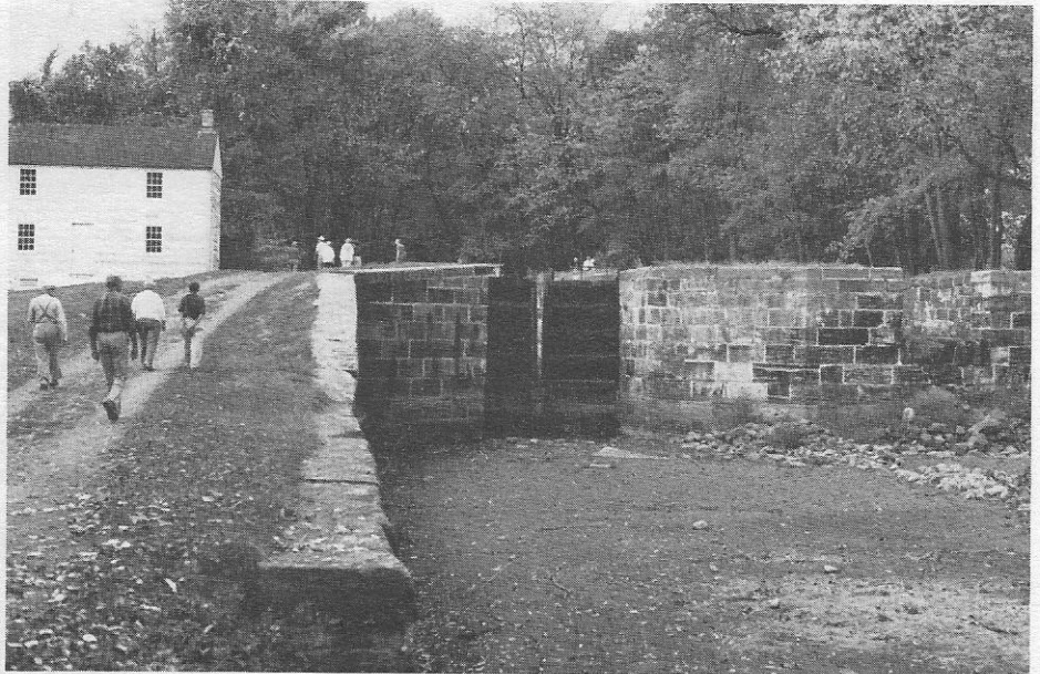
One of the locks at Oldtown, with a log lockhouse at the left. There is no water in the canal at this point, but the rebuilt lock gates are still in good shape. Note the bypass flume to the right.
