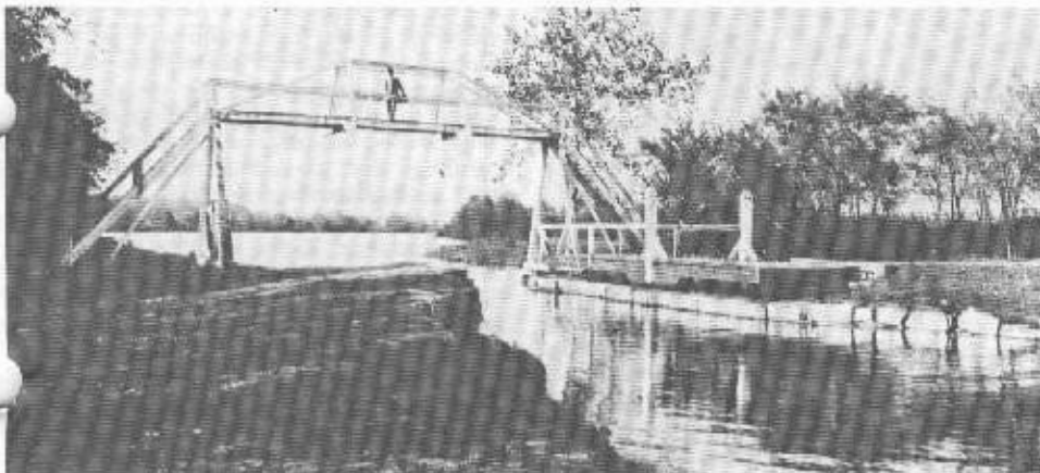
Pedestrian bridge and pivot vehicle bridge on the Chesapeake and Ohio Canal at Stop Lock, Ft. Frederick, Maryland. Circa 1910. (Courtesy National Park Service.)
