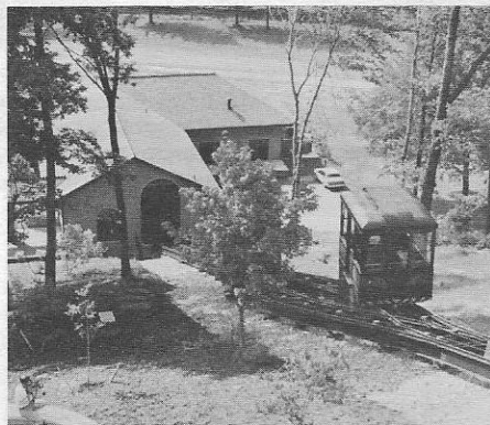
Looking down from the Horseshoe Curve at the new Visitor's Center. The Inclined Plane can be seen at the right, carrying visitors between the upper and lower levels. The cars are completely automatic and use a single track, with a turn-out at the half-way point.
