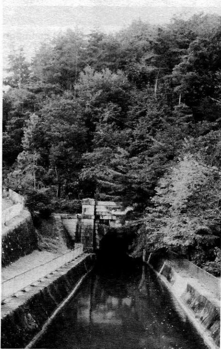
Looking west from the pedestrian bridge to the east portal of the third tunnel.
