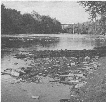
Photo, made by W.R. Smith in 1941, of the remaining keel and ribs of canal barge just below the C. & O. Aqueduct across the Monocacy River.
