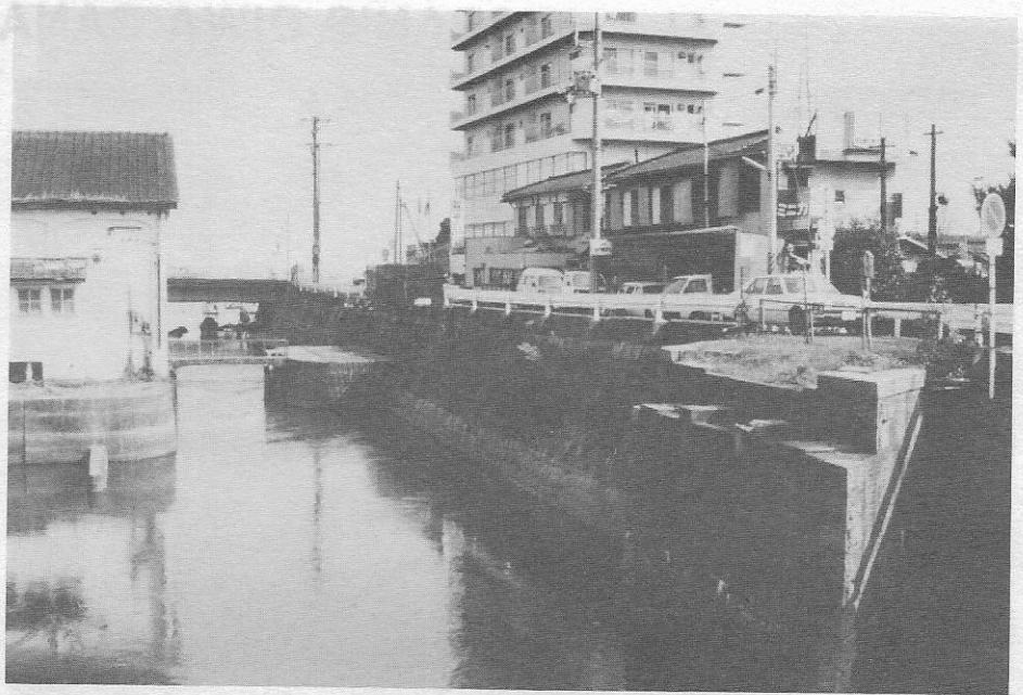
The entrance to the Lake Biwa Canal, looking east from a street bridge in Otsu. Lake Biwa is in the background. The guard lock shown is apparently no longer in use; the bridge abutment is from an abandoned railroad.
