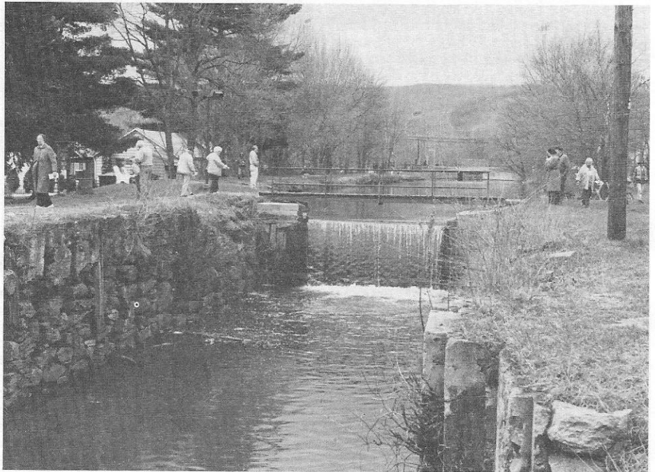
Restored section of the Lehigh Canal At Walnutport. A weir has replaced the upper lock gates.
