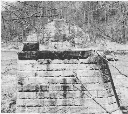
Portageville Aqueduct Site —Having completed its diversion to the east side of the Genesee River to bypass the Letchworth Gorge, the GVC crosses over to the west side again over a 7 span, wooden trunk aqueduct 50 ft. above the river. The abutment on the far side is preserved unchanged from the canal era. The piers in the foreground are remnants of the RR trestle that replaced the aqueduct.
