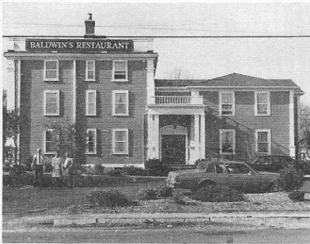
The Baldwin Mansion (now a fine restaurant) was the site for our dinner after the annual meeting of the Middlesex Canal Association. The Baldwin House was the home of Loammi Baldwin, Chief Engineer for the Middlesex Canal.
