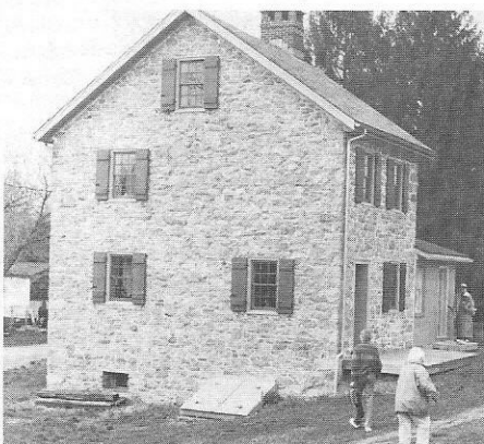
Restored lock-house at Walnutport.
