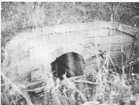
Small Culvert —A well preserved 4 ft. arch culvert a few miles south of Mt. Morris, NY. The Canal Prism is readily visible here for several miles paralleling NY Route 36.
