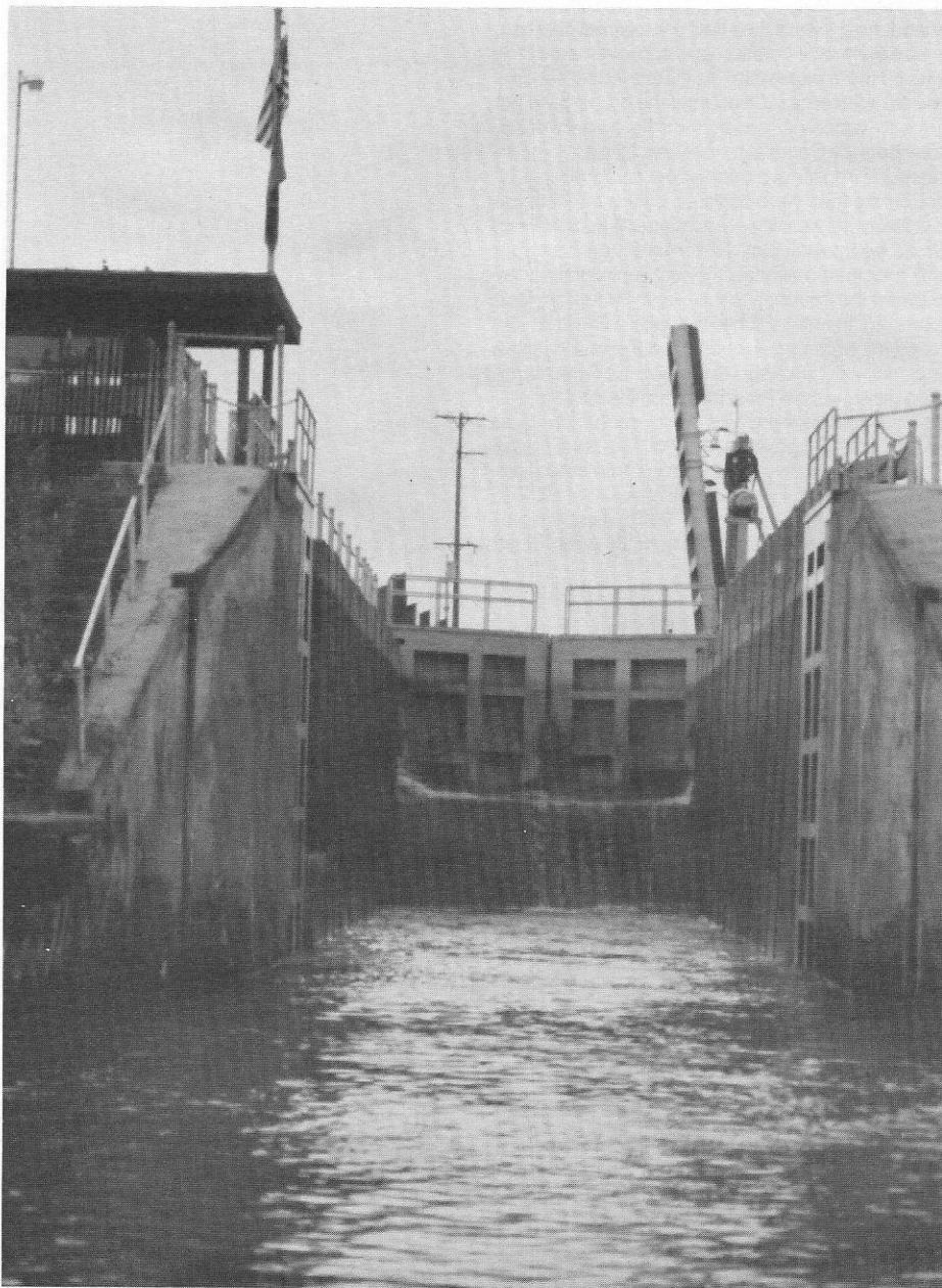
The Cheboygan River lock, open to receive upbound traffic.
