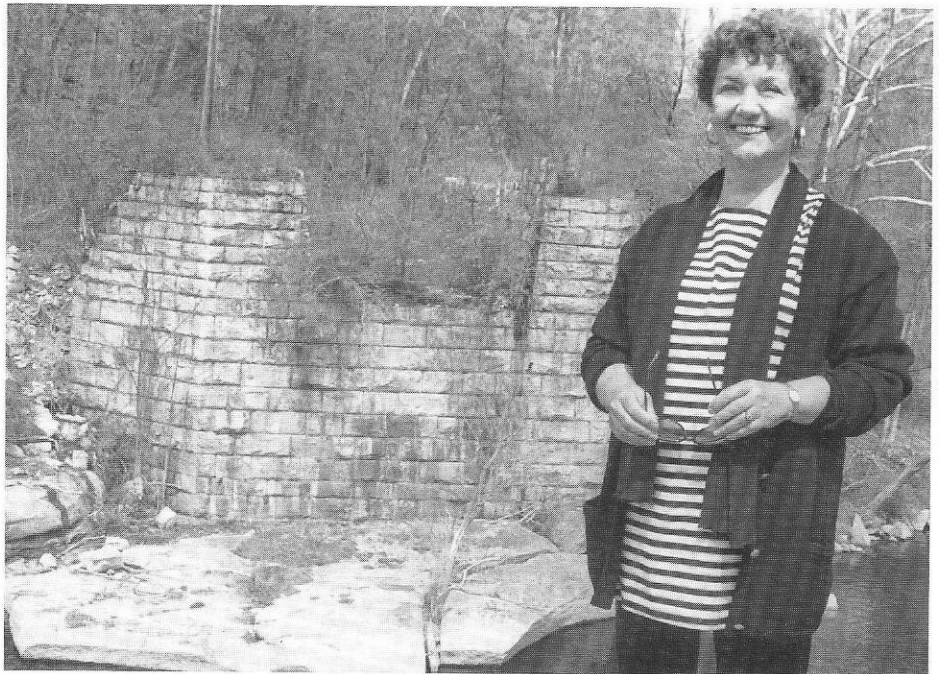
Mary Cassai poses on the lip of the High Falls south abutment of the John Roebling Suspension Aqueduct — the second aqueduct to be built at that point.
