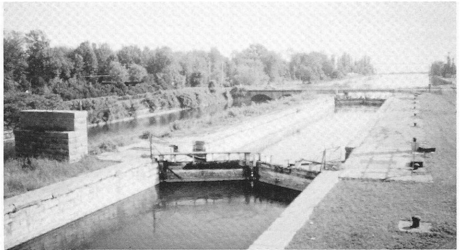
Soulanges Canal. View of Lock 5, looking west from railroad swing bridge.
