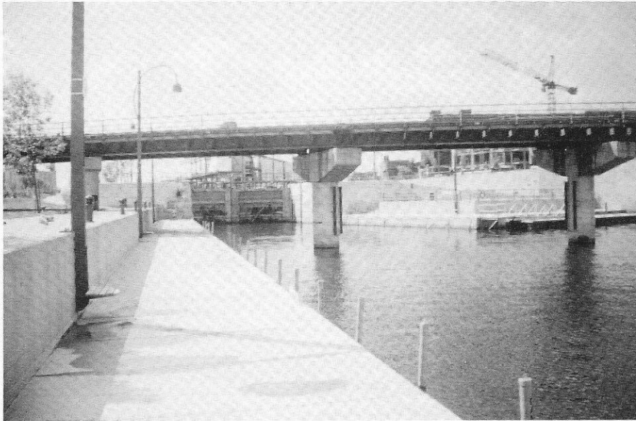
Lachine Canal. Lower distant view of Lock Number 1, north chamber.
