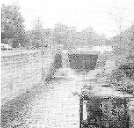
Soulanges Canal. Lock No. 1, looking west.
