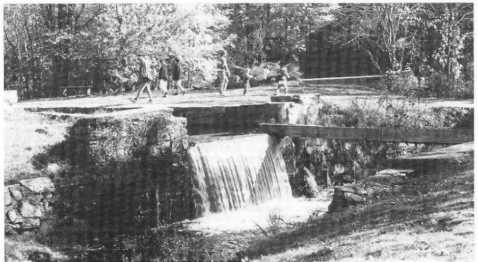
A spillway on the Morris Canal in Waterloo Village, at the foot of an inclined plane. A small wooden flume carries some of the water to the next canal pool.
