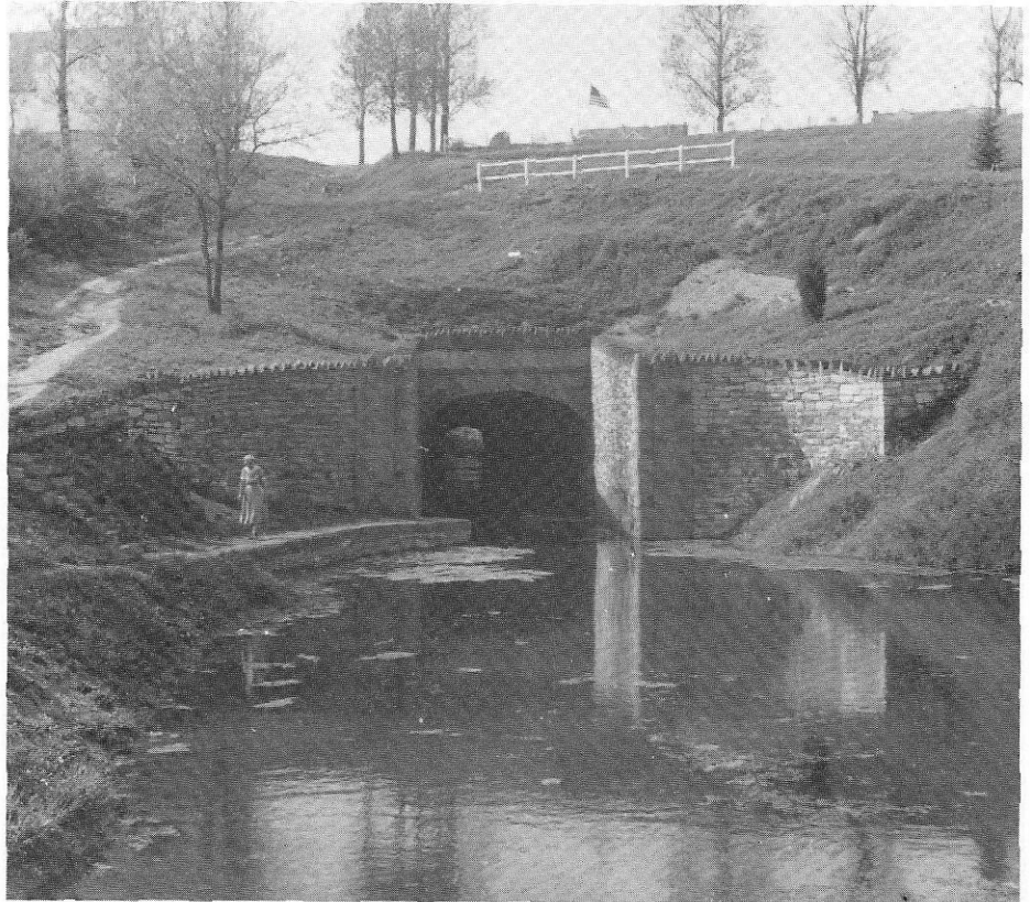
The Union Canal Tunnel (south portal) on a 27-acre tract owned and maintained by the Lebanon County Historical Society. The mule team climbed over the hill, while canal boats were poled through the tunnel. Traffic ceased in 1885, due to the difficulty of maintaining water in the upper reaches of the canal, and the competition of the railroads. (Photo by Bill Shank)
