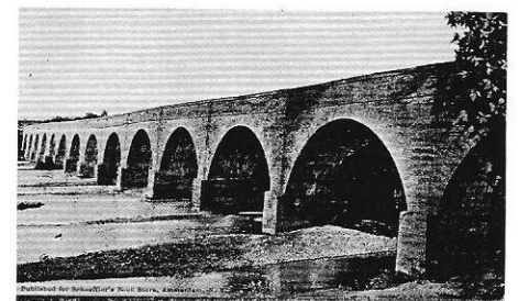
Aqueduct that Carried the Old Erie Canal Across Schoharie Creek at Fort Hunter.
