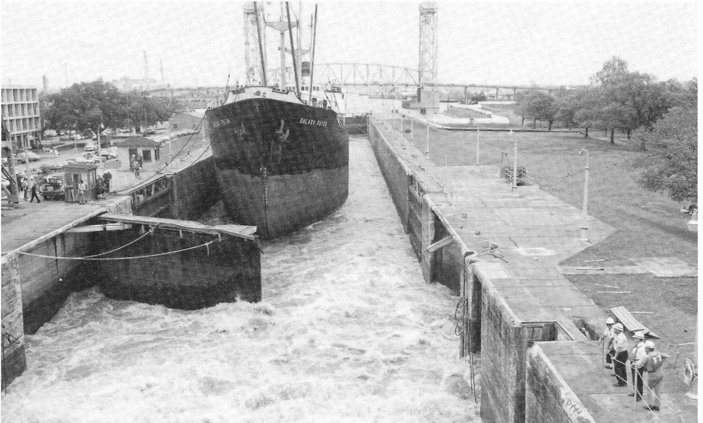
A "Great Canal Disaster" occurred when The GALAXY FAITH struck the upper gate of the Inner Harbor Navigation Canal Lock in New Orleans on April 5, 1972, closing the lock for 18 days. Fortunately for the GALAXY FAITH, her adventure was less exciting than the ASSINIBOLA's record-breaking trip through a lock in 1909. (Photo courtesy of the New Orleans District, Corps of Engineers)
