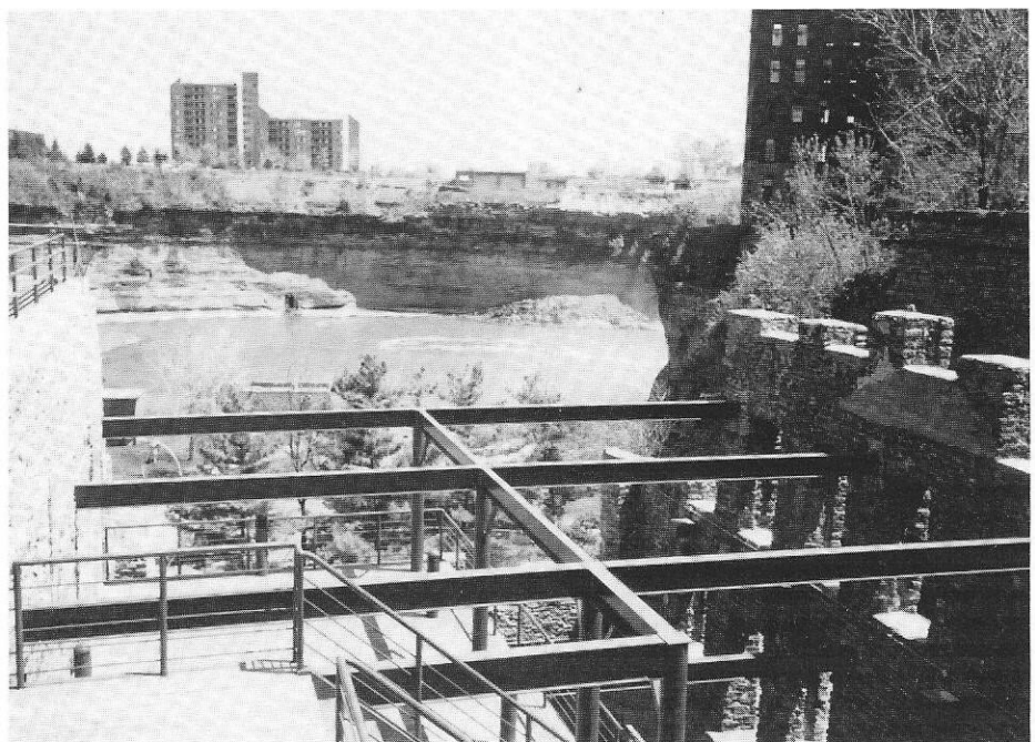
The ruins of one of the many factories lining the sides of the Genesee River Gorge in Rochester. All depended on the hydraulic water "head" for power. This particular ruin is all that remains of a trip hammer forge. (Russell photo)
