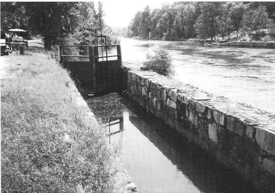
Augusta Canal Headgate Lock.
