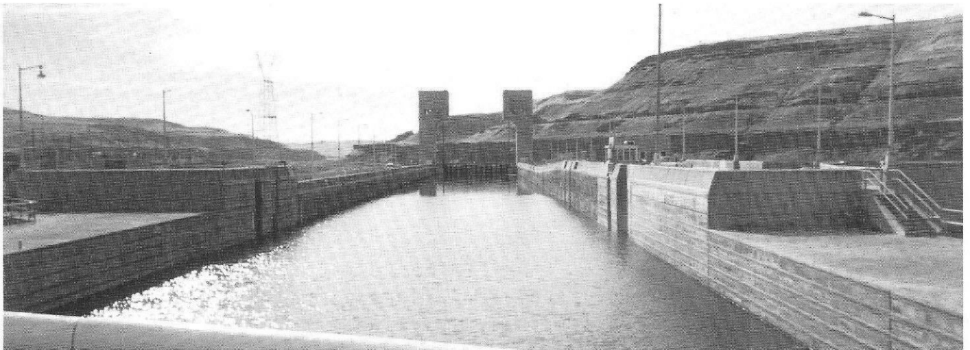
A typical lift-lock on the Snake River as seen from the upper entrance. Note the Guillotine Gate in the closed position at the opposite end. The landscape is typical of the scenery east of the Cascade Mountains. We passed through some of the highest lift-locks in the world on our journey.
