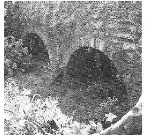
Rae's Creek Aqueduct, with its double-arch opening. Masonry in excellent condition.
