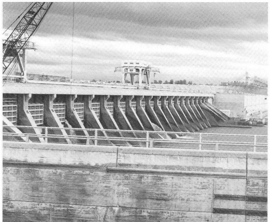
McNary Dam as photographed from the north-side lift-lock.
