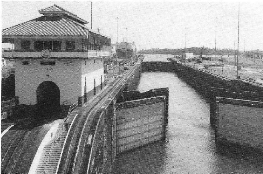
Looking backward as we leave the upper lock at Gatún, with the Lake in the distance. Note the double lock gates closing behind us, a safety feature to assure the level of the lake water.
