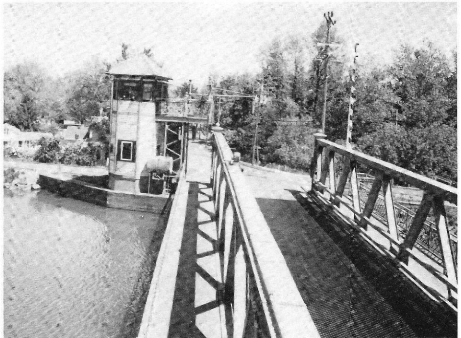
A close up of one of the many lift bridges on the western section of the canal, in "down position". The operator sits in the control tower shown and raises the bridge when a vessel passes. The operation is a necessity, since most of the bridges barely clear the water when conveying highway traffic across the canal.
