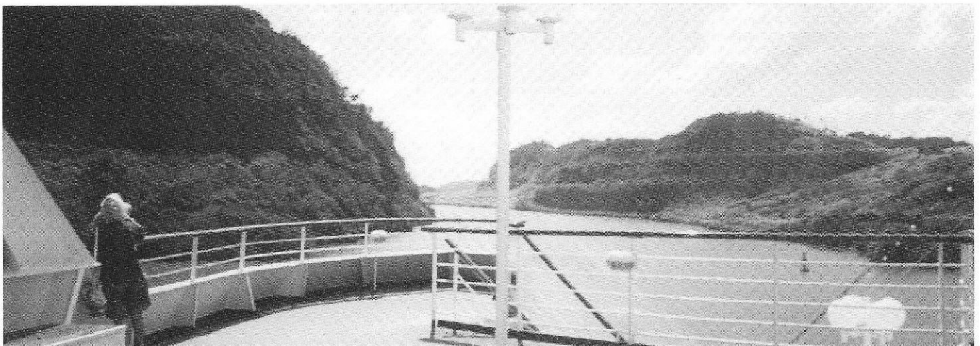
We pass through the Culebra Cut, where the most difficult excavation work took place on the Canal. Cave-ins and slides developed here, both during construction and afterward. Today there is still a continuing operation to widen and improve the banks of the "cut".
