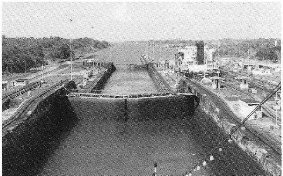
Lower gates of the three Gatun Locks as our boat drops from the level of Gatun Lake down to the Atlantic. Like all locks on the Canal, the locks are double and a large freighter is being towed downstream in the lock parallel to ours.
