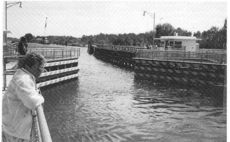
W.P. Franklin Lock, Upper Gate Closing, Okeechobee Waterway Florida.
