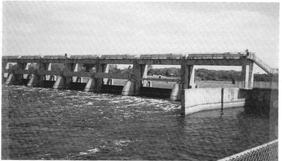
The W.P. Franklin Dam, Okeechobee Waterway, Lee County Florida.
