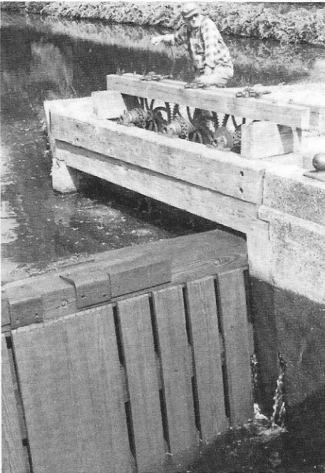
A lock attendant cranks up the special drop-gate designed by Josiah White, on the lower Lehigh Canal, after our canal boat passed through.
