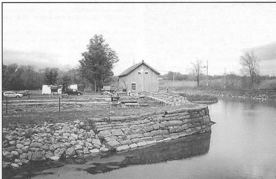
View of the rebuilt general store alongside the Erie Canal and entrance to the launching basin.
