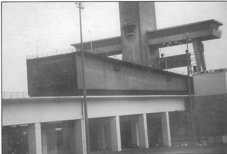
Caisson at upper end of Ronquieres inclined plane, Canal Charleroi, Belgium
