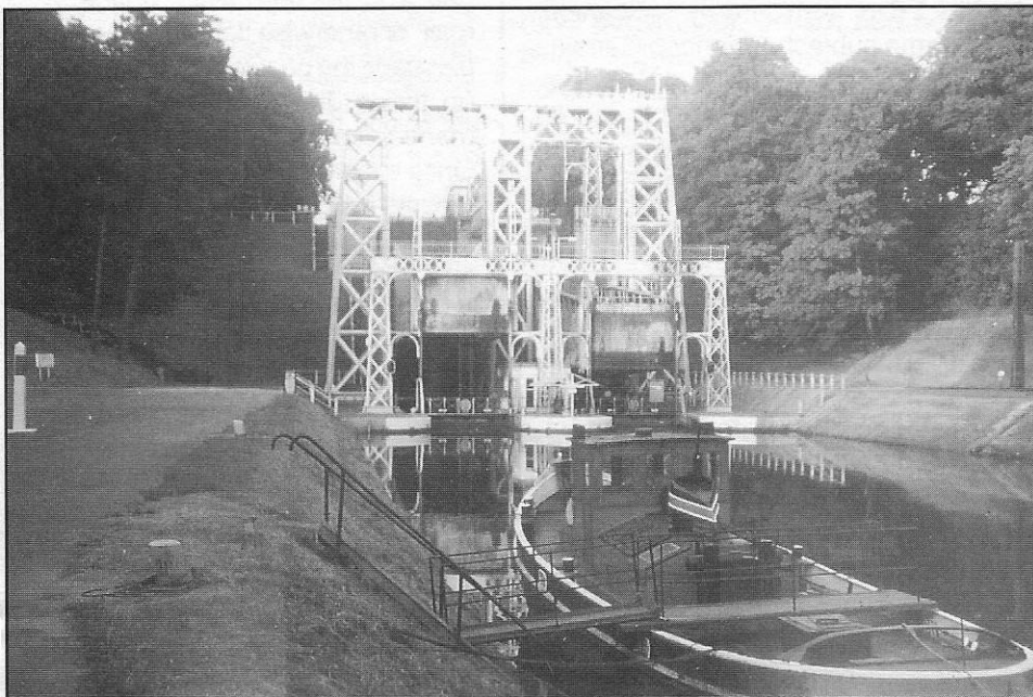
Hydraulic lift #3 on the old 350-ton waterway, Canal du Centre, Belgium
