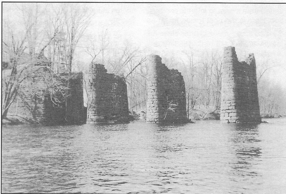
Piers and abutment of the Farmington Canal aqueduct crossing the Farmington River
