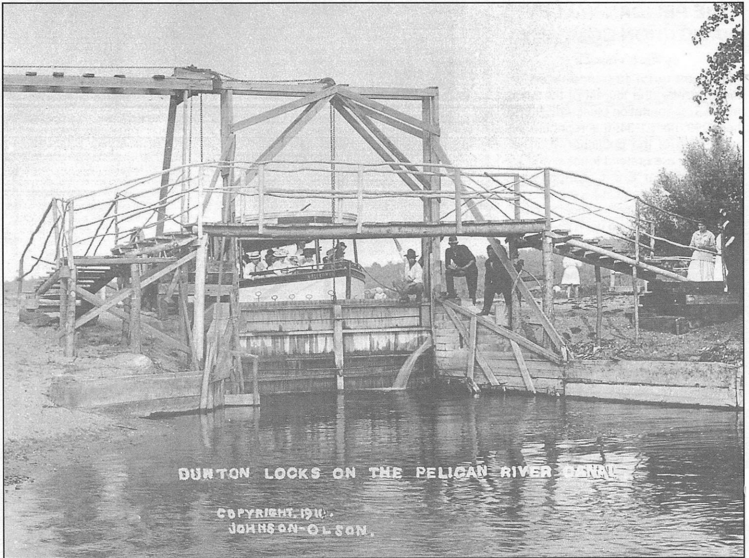
Mayflower being lowered at Dunton Locks. All locks on the waterway had guillotine gates.
