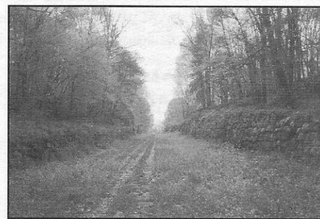
View from about mid-point of the inclined plane. Some of the stone rail bed, as well as the stone retaining walls can be seen.
