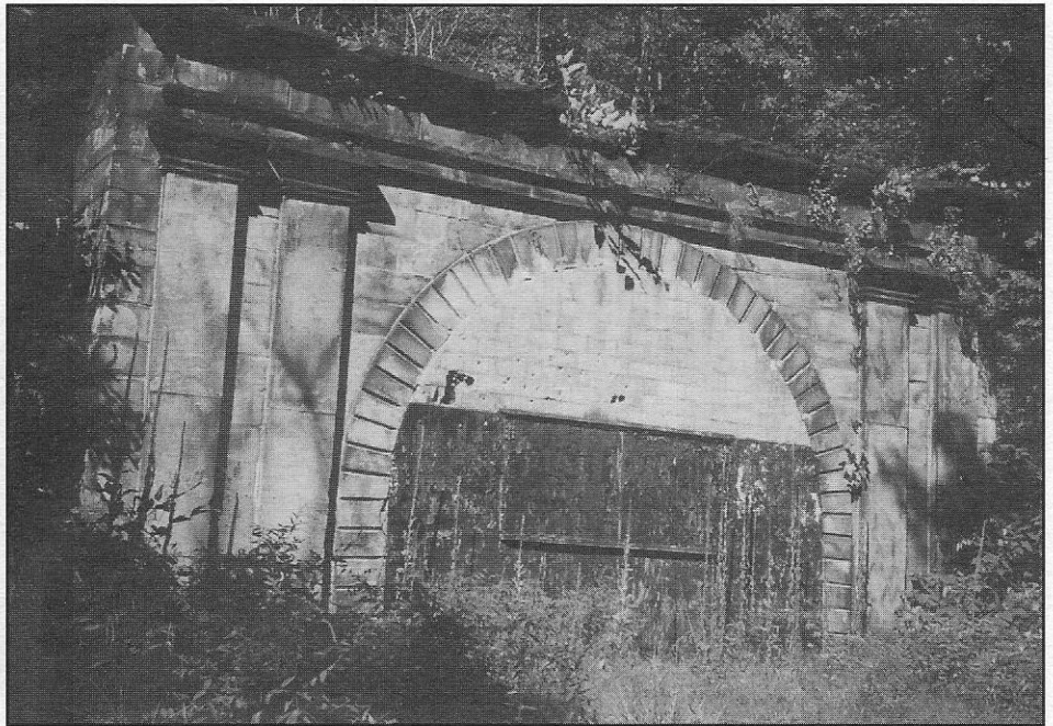
The western portal of the Staple Bend Tunnel before restoration.
