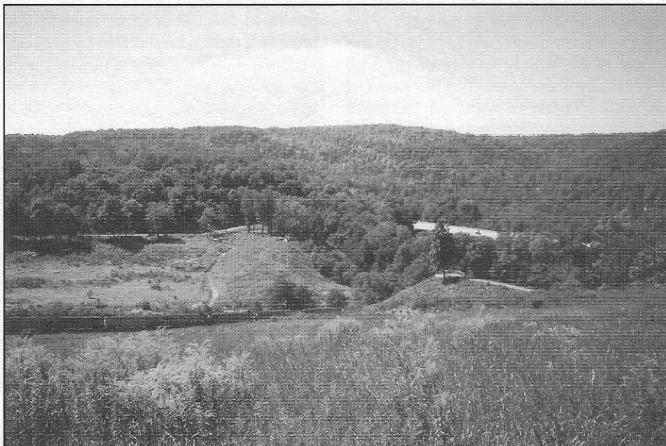
The two mounds which anchored its ends are all that remains of the South Fork Dam. A railroad train passes through the gap between them.
