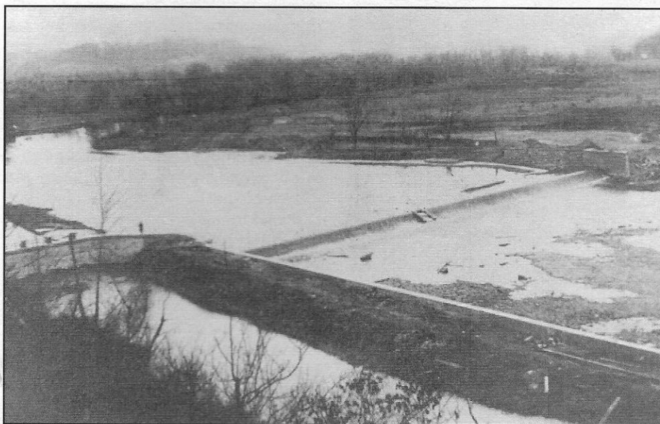
Six-Mile Dam on the Walhonding River, and the Walhonding Canal (on left, with head-gates) after 1909 reconstruction.
