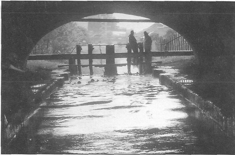
A Royal Canal lock under a stone bridge in Dublin.
