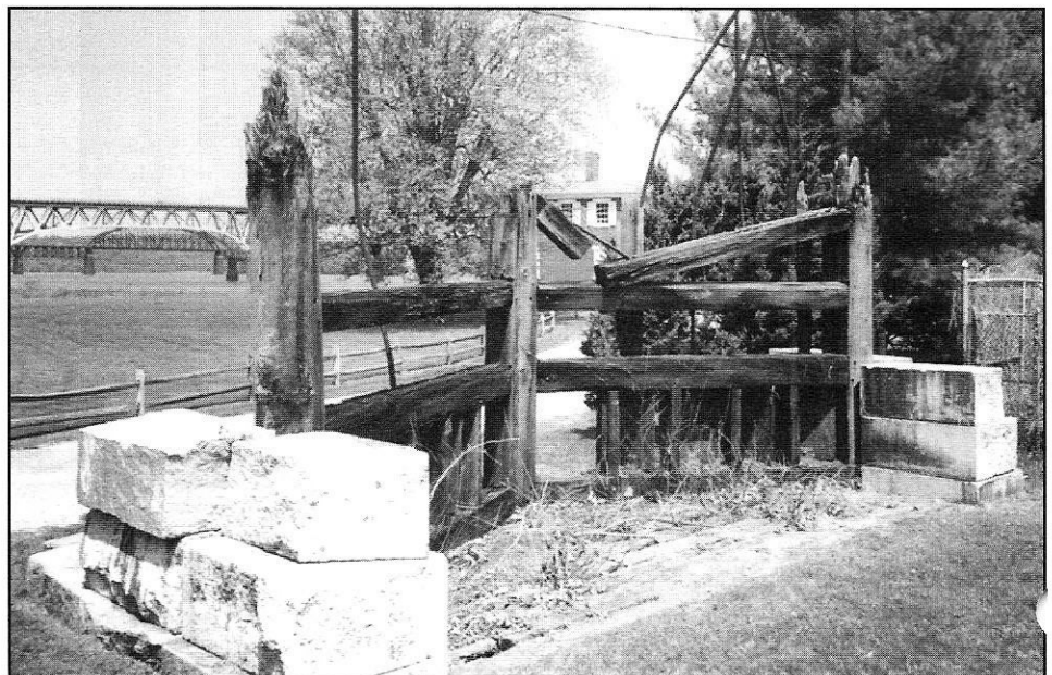
The remains of one of the wooden lock gates on display on the grounds of the lock-tender's house
