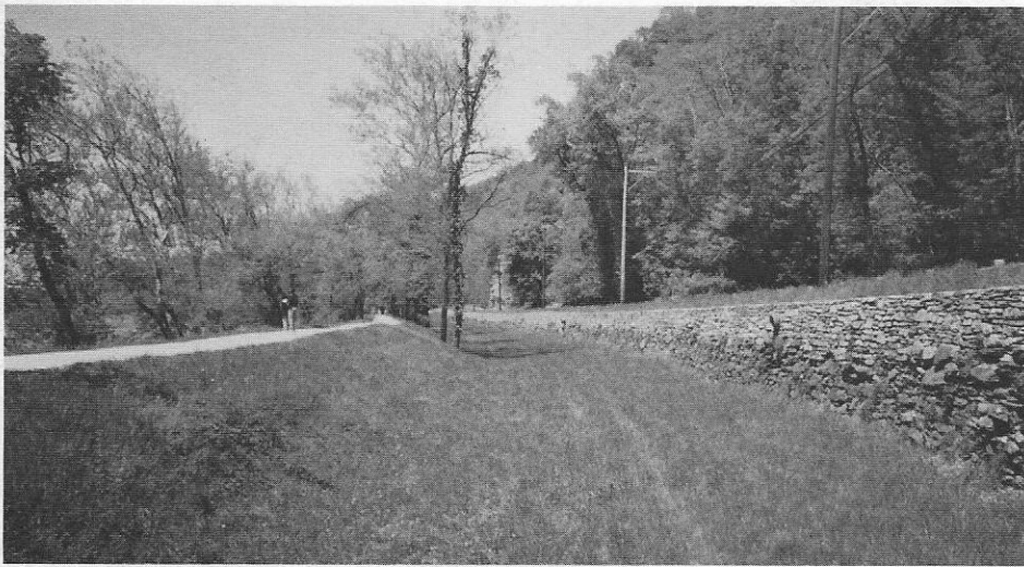
C&O Canal, opposite Harpers Ferry. Restoration of the towpath and the retaining wall is finished. All that's missing is the 4-5 feet of water. Photo by Bruce Russell, April 2001.
