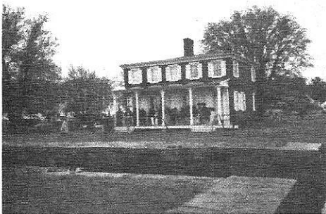
The Lock House and outlet lock of the Susquehanna & Tidewater Canal, Havre de Grace, Maryland. Photo by Robert H. Barth.
