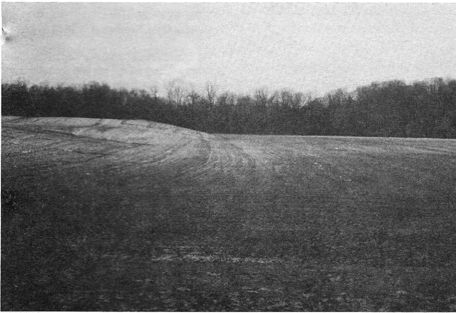
Very faint trace of the feeder channel as it curves through old corn field from the dam toward Ohio Canal. This area is now a gravel pit. Photo by Terry Woods.
