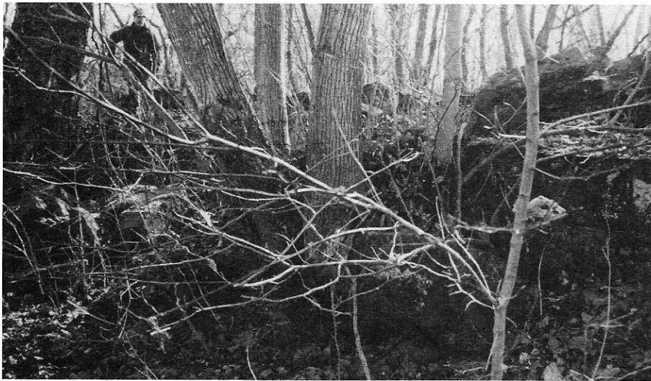
Remains of right dam abutment to feeder dam in Walhonding River. Photo taken in 1994 by Terry Woods.
