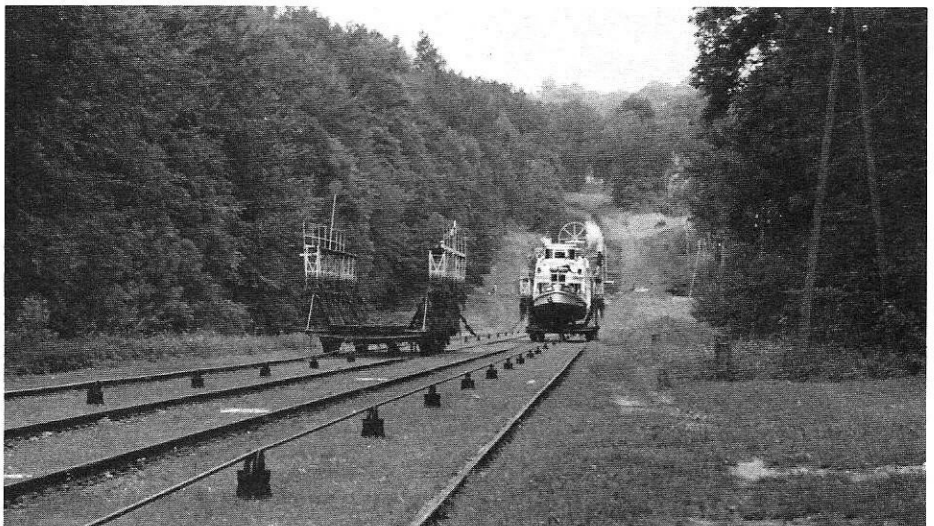
Looking down Plane 5 on the Elblag Canal. The empty cradle car, heading down, is about to pass the loaded car. Photo by Linda J. Barth
