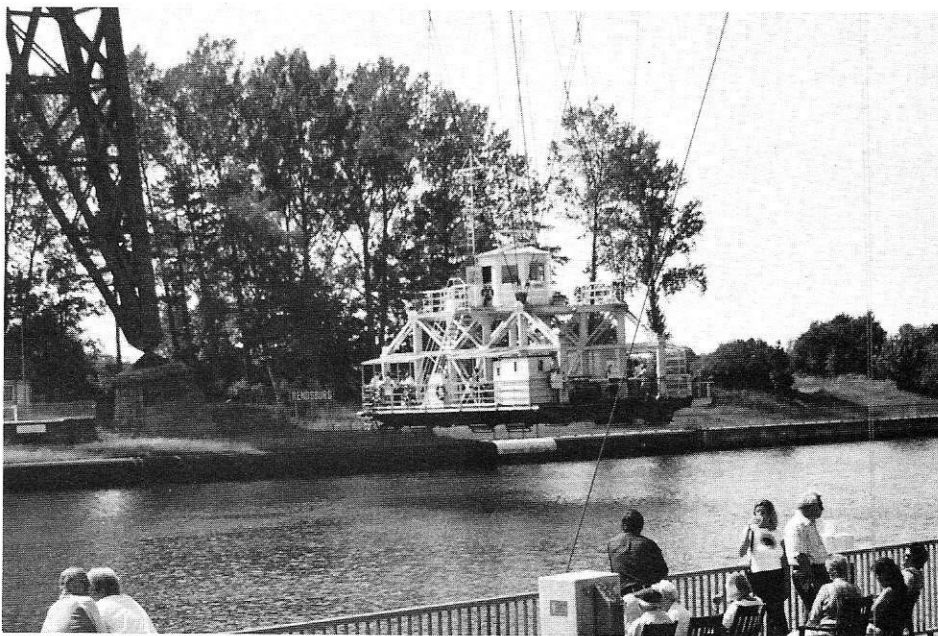
A transporter ferry, suspended from the bridge by cables on a trolley, takes cars and passengers across the canal, just above water level. Photo by Linda J. Barth
