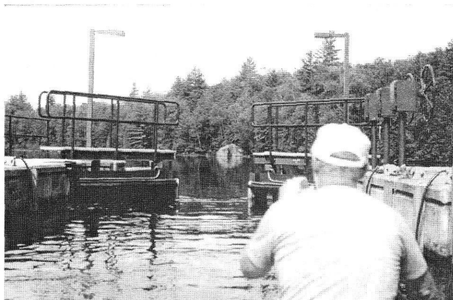
On exiting the lock, you pass the manual control wheels used when the lock tender is not on duty. Two of the wheels control the gates and the third controls the valve.
