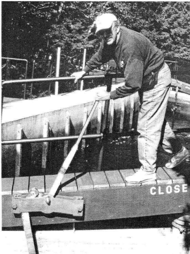
The author, working a valve lever on the gate. Photo by David Kipp
