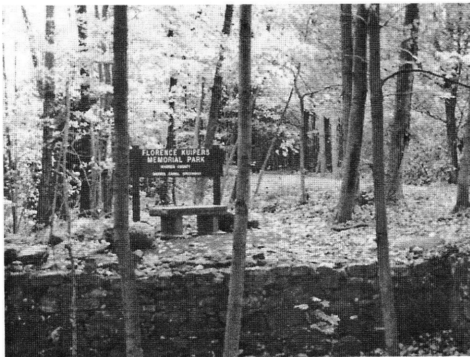
Foundation of the canal store in Florence Kuipers Memorial Park.
