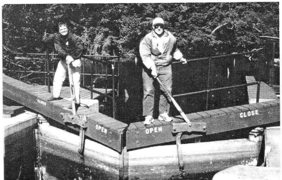
Canal Society of NY State member Carl Brozek and friend Jack Redfield man the gillotine valve levers built into each of the four gates. Photo by David Kipp
