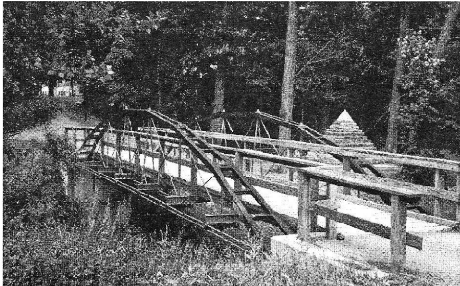
Photograph 7: Whipple Bridge on Union College Campus, Schenectady, NY
