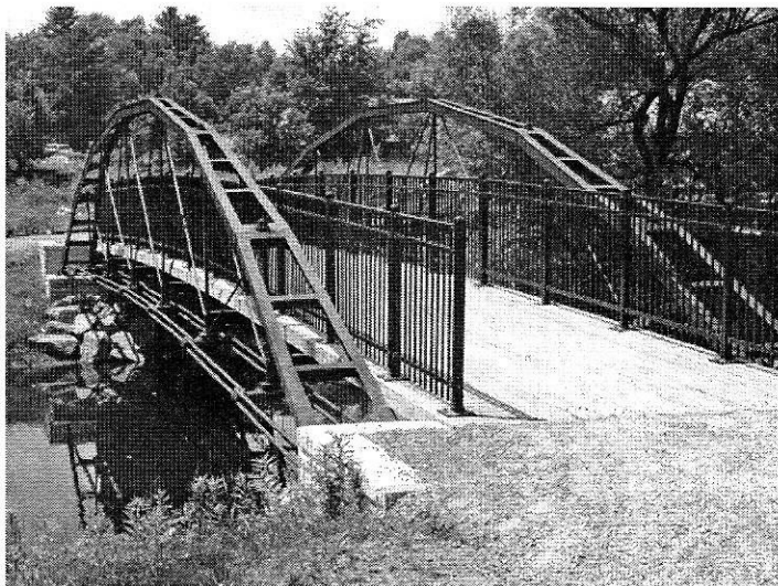
Photograph 9: Boonville, NY Whipple Iron Truss Bridge
