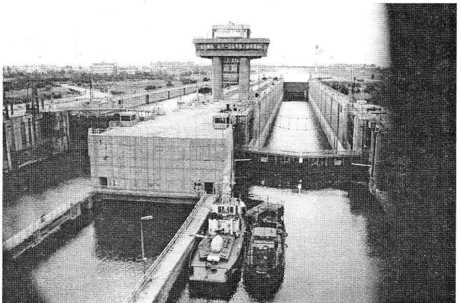
Lock at Agigea, looking west from the railroad bridge. Note the highway bridge beyond the end of the lock.
