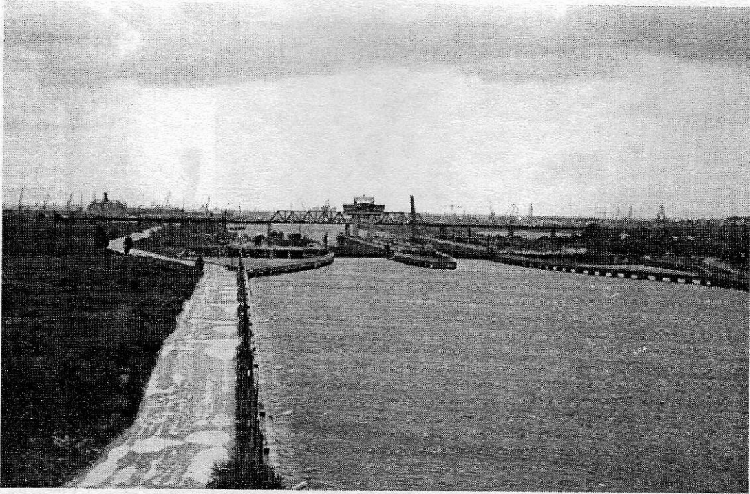
Lock at Agigea, looking east from the road bridge. Note the railroad bridge beyond the east end of the lock.
