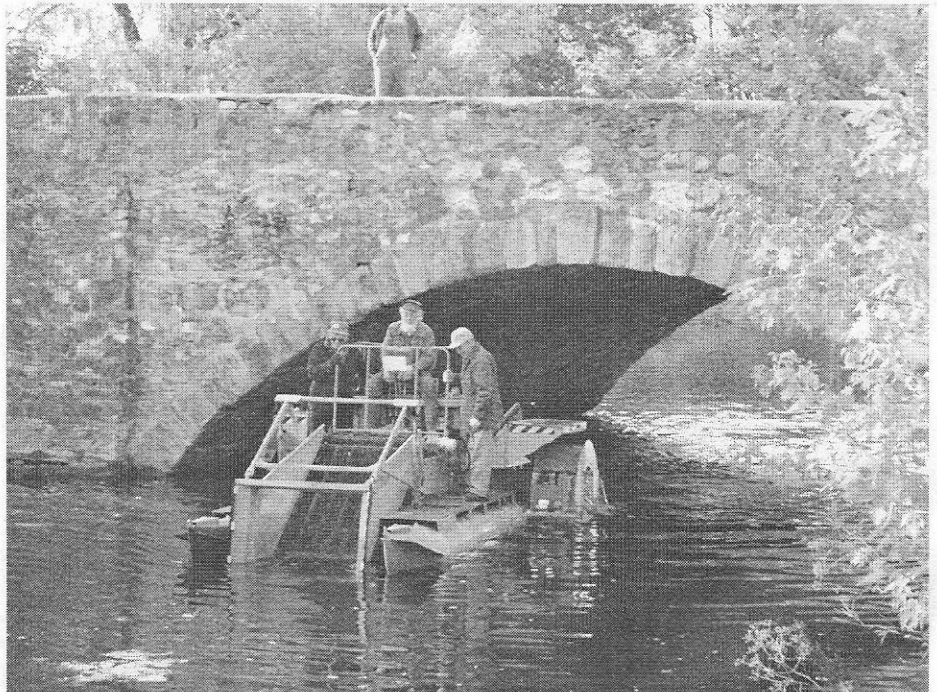
"Clean Mary II" with the cutter head in the down/operating position as she passes under the 1901 historic stone arch bridge.
