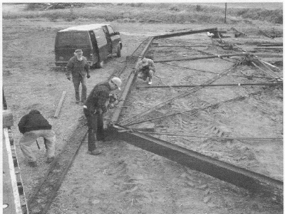
The disassembled bridge components are laid on the ground.
