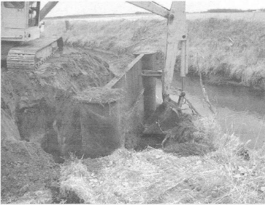
Removing soil from the unusual metal caisson foundations.
