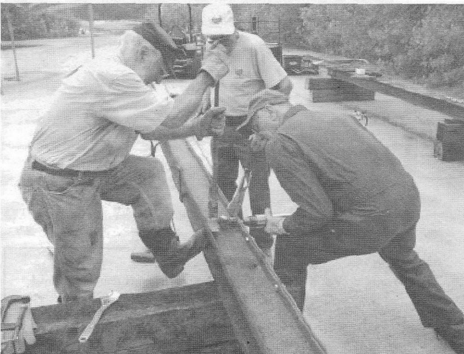
Volunteers replacing missing and broken rivets.
