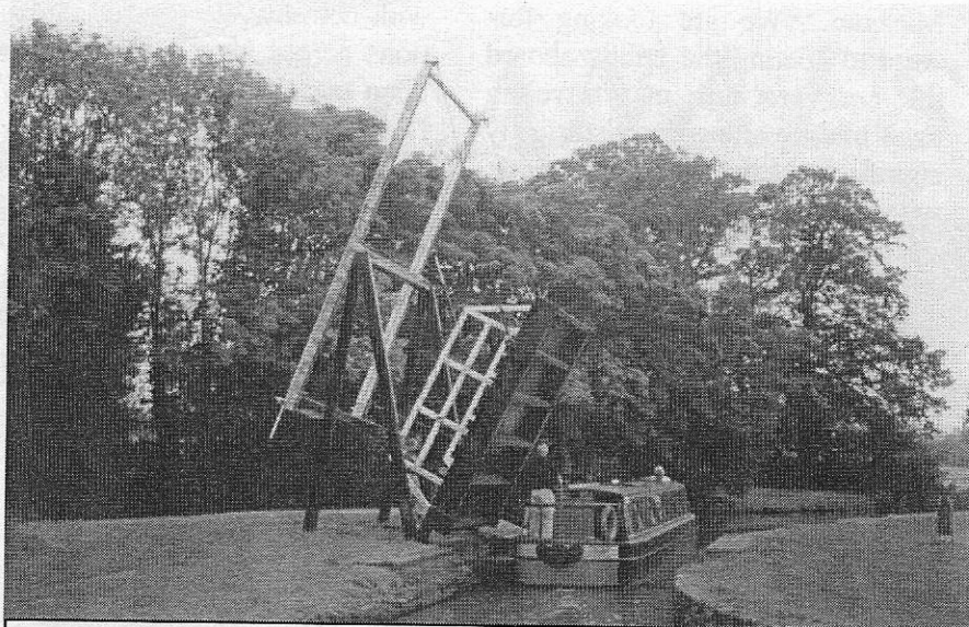
One of the many lift bridges under which we passed. One of the crew disembarks, runs ahead, and cranks the bridge open. Photo by Bruce Russell
