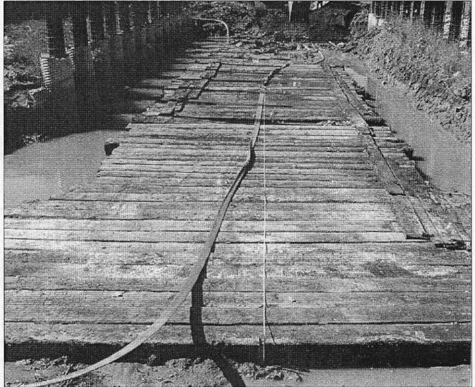
Cross cut culvert 151, Terre Haute, Indiana
