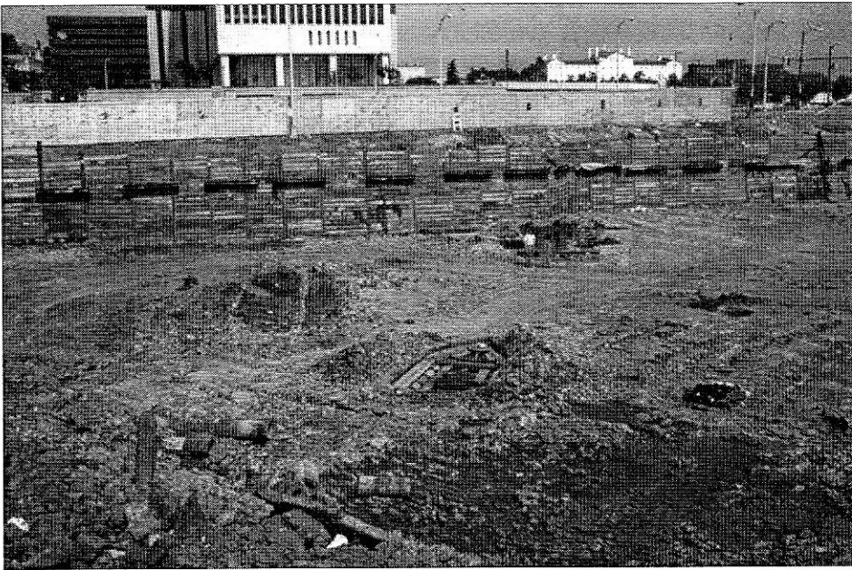
A view from inside the Richmond Canal Basin dig.
