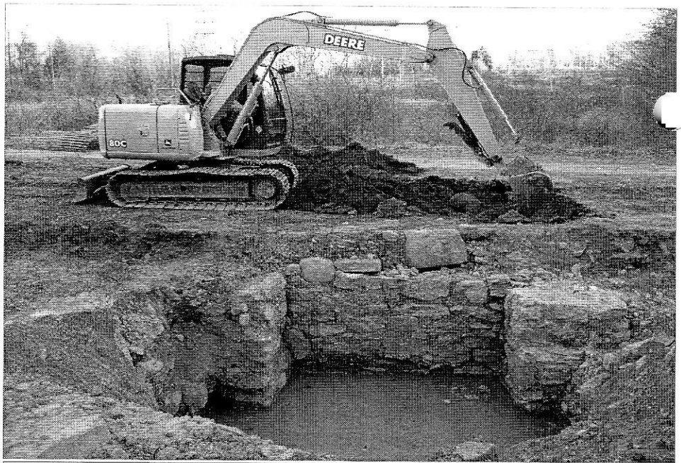
The outside face of the south lock wall has stone buttresses that protrude from the face of the wall. These allow a thinner wall between the buttresses.
